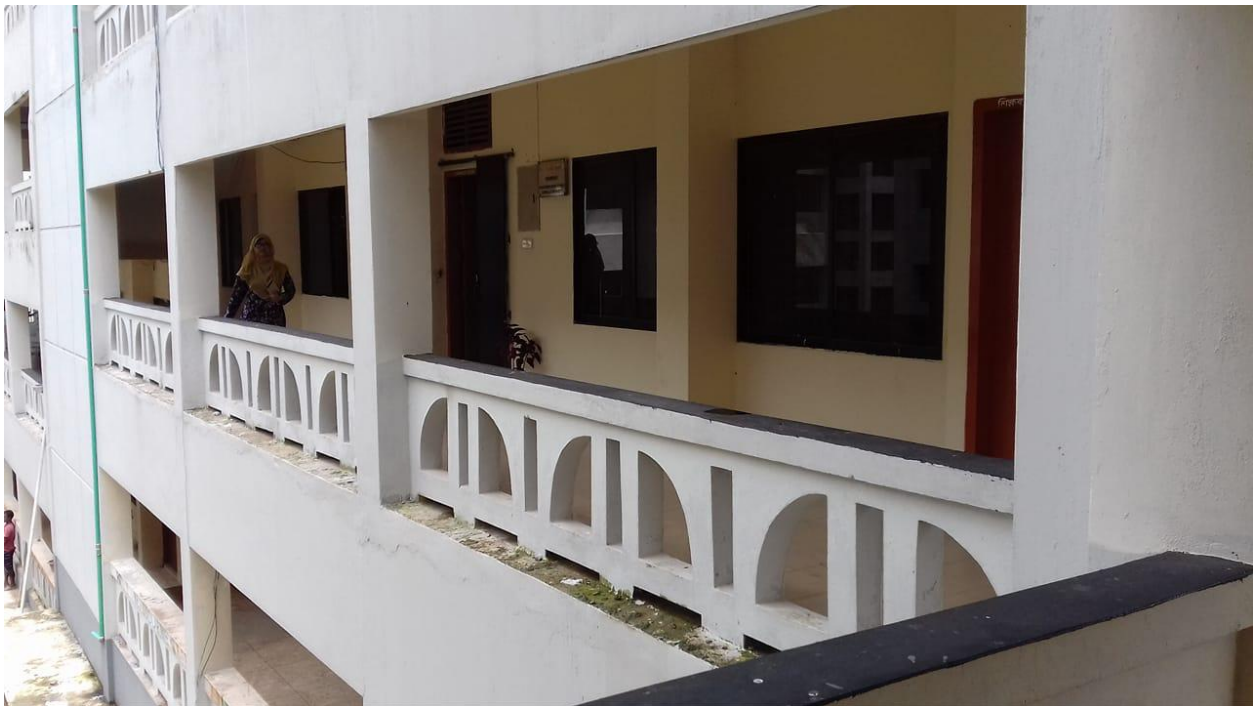
Corridor (2 nd floor)
