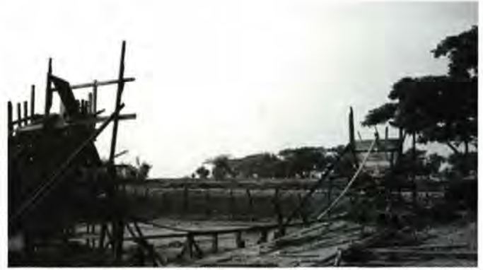
Fig. 4.12 The laying of the keel, stem and sternposts of a ship, Sandwip
