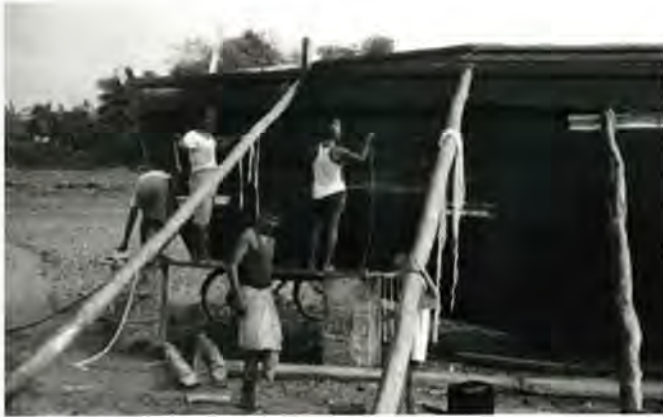
Fig. 4.15 A Kalpat Mistri inserting cotton thread for chaulking a ship, Sandwip
